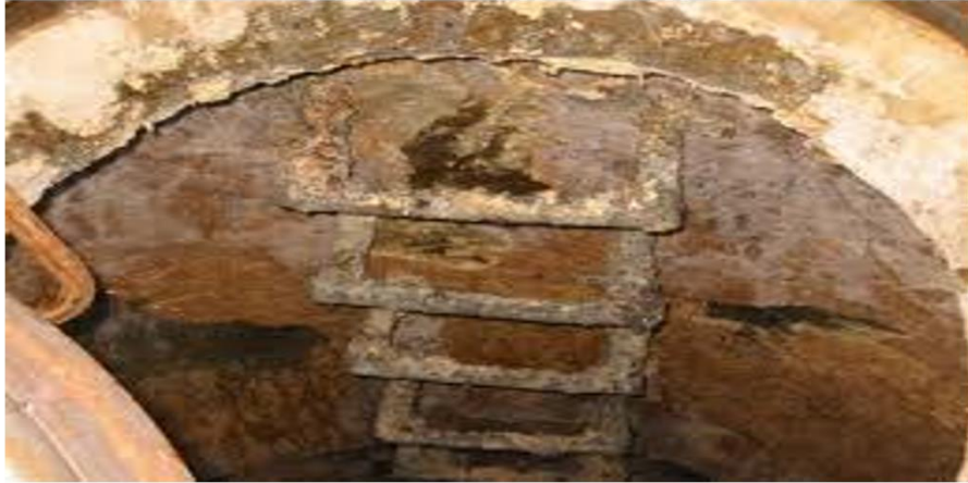
Corroded stair treads
