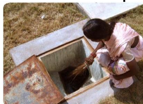
Cleaning of inspection chambers
