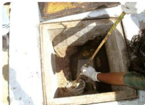
Removal of obstacle from the sewer pipeline
