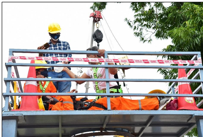
Figure 8: Procedure for first aid post retrieval of persons from sewer maintenance hole
